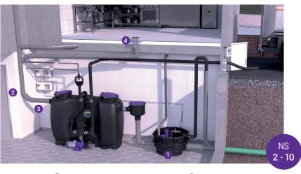
1 Properly sized hybrid lifting station 3 Wastewater calming section
