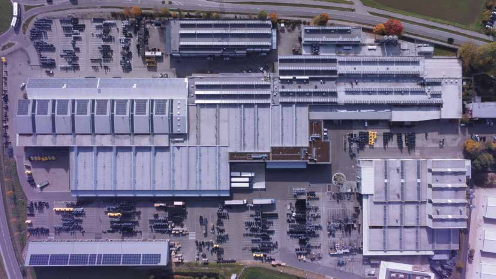
KESSEL Headquarters Lenting, Germany
