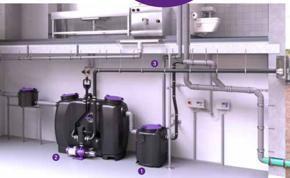
1 Lifting station 2 Grease separator 3 Pressure pipe
